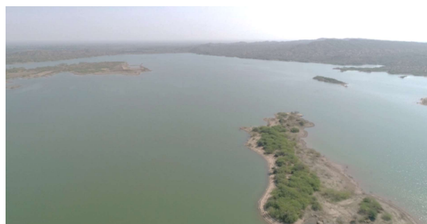
Figure 3. Larger sites, such as Nara Dam, required drones for effective surveys.
